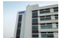
Newly constructed technical center in China
