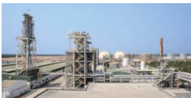
The Phu My Plastics and Chemicals plant, the latest new production base after Thailand and Indonesia
