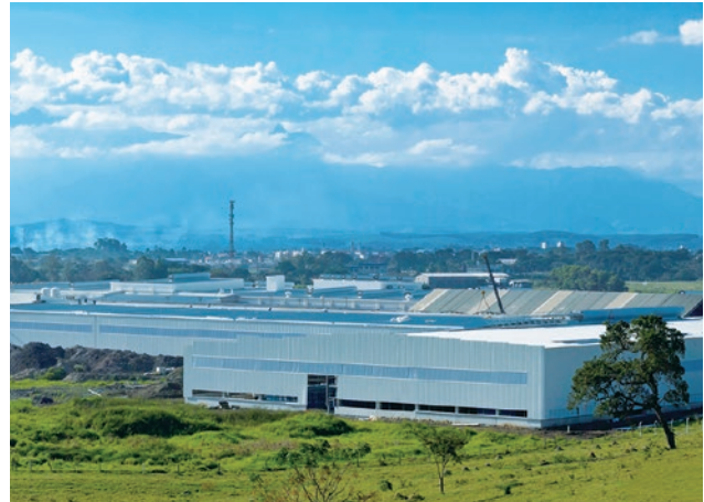
AGC Glass Brazil plant
