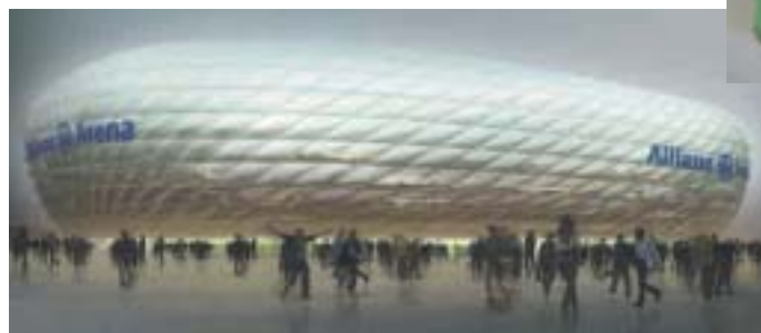
Fluon™ ETFE film will be used in the construction of the Allianz-Arena soccer stadium for the 2006 World Cup in Germany
