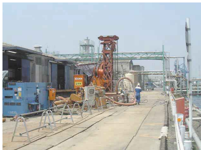
Impervious wall installation work at the Chiba factory
