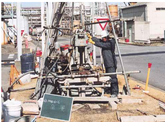
Soil survey by boring at the Chiba factory
