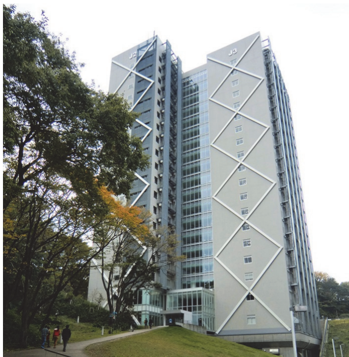
J3 Bldg., Suzukakedai Campus, where the Collaborative Research Center will be set up
