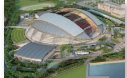
National Stadium's roof using Fluon®ETFE Film
